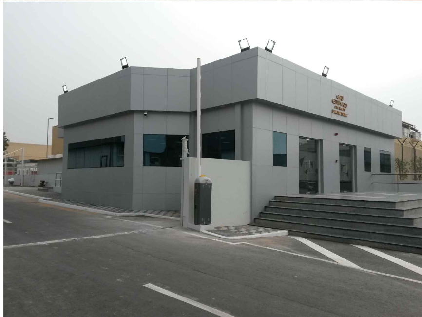
Etihad Airways Engineering Security Buildings, Abu Dhabi For Al Etlala General Contracting, Abu Dhabi
