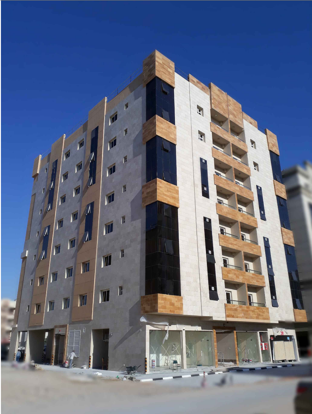
B + G + 7 Floor building, Moweilah, Sharjah For Al Mudhafar Building Cont. L.L.C, Sharjah
