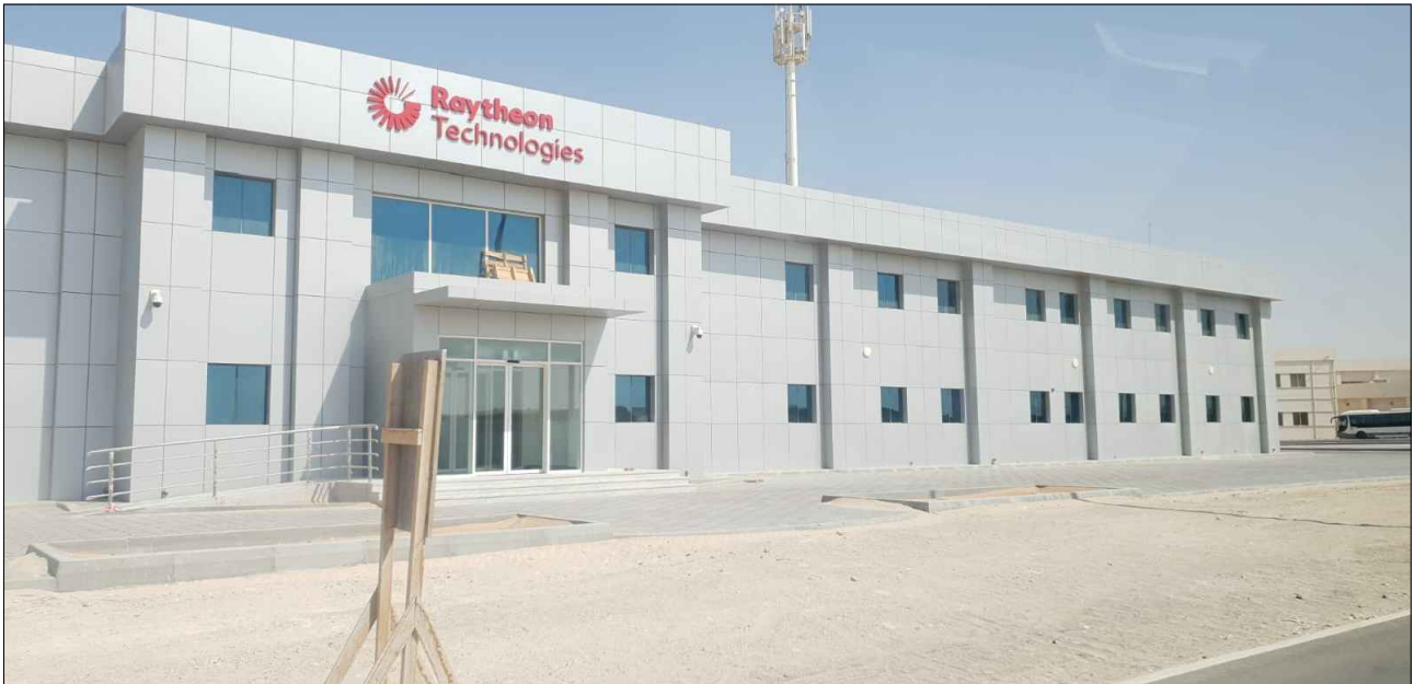
Design and Build of Modular Office Complex, Zone 3 at Tawazun Industrial Park (TIP) Ajban, Abudhabi- UAE, For JAZAL Building Engineering LLC.
