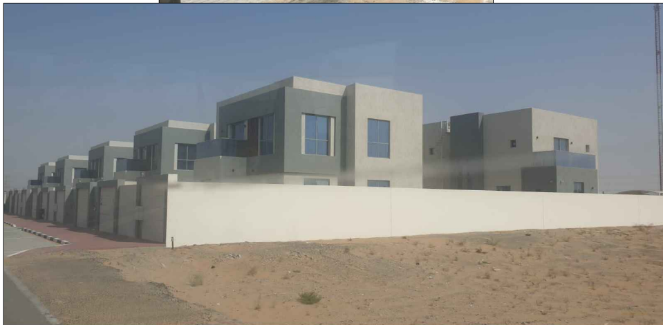
20 VILLA EASTERN SECTOR, AL HELIO, AJMAN
