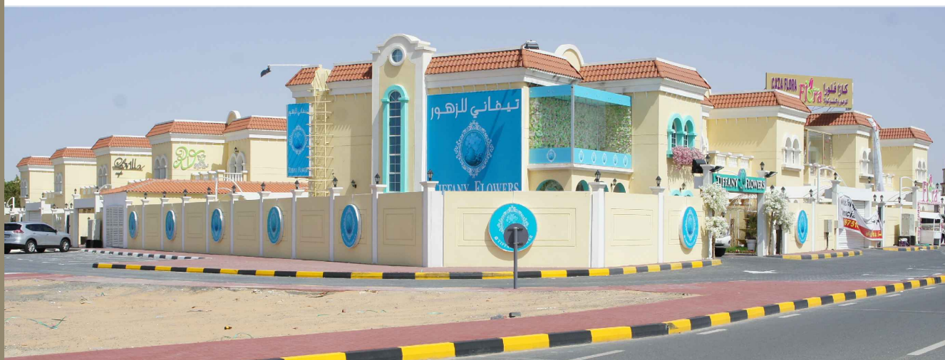
8 Villas, Al Juruf, Ajman For Al Zamalek General Contracting L.L.C, Sharjah
