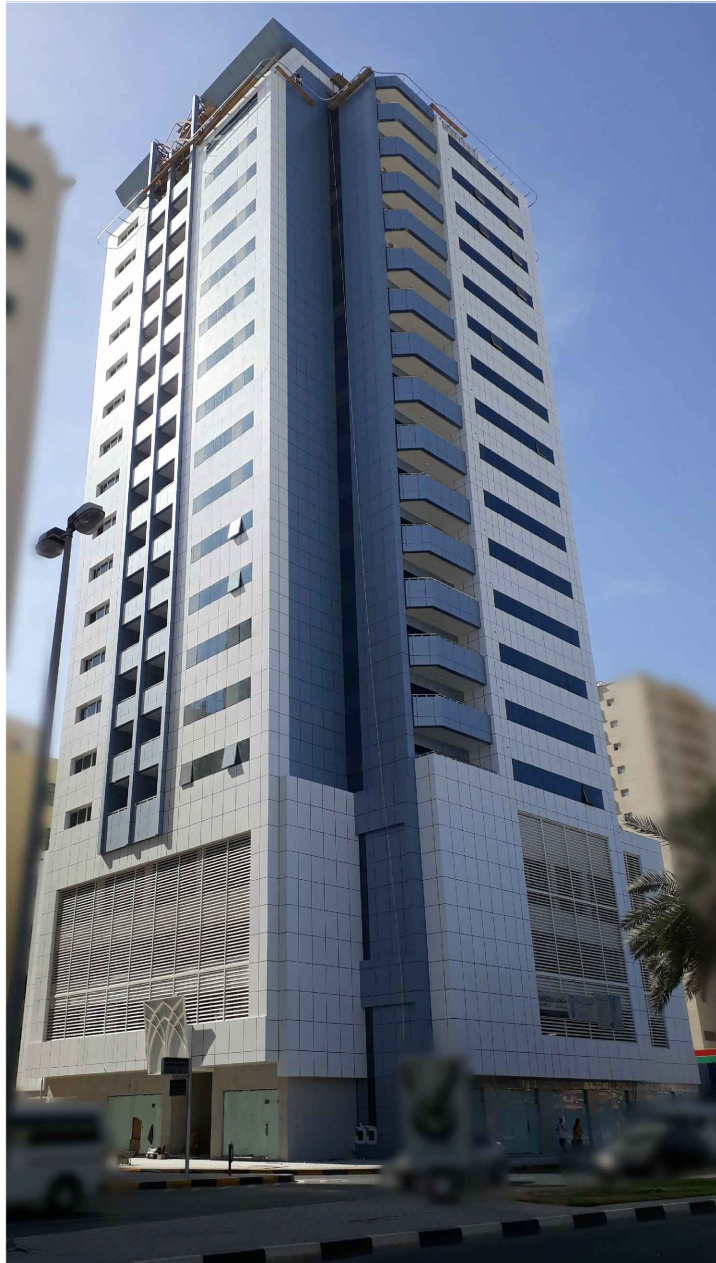
G + 3P + 15 Floors Building, Al Mahatta, Qasimia, Sharjah For Sarco Building Contracting L.L.C, Sharjah
